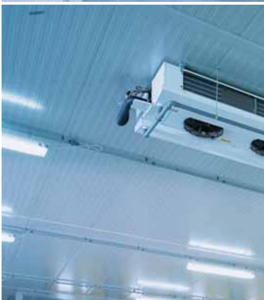
Detail of the internal side
